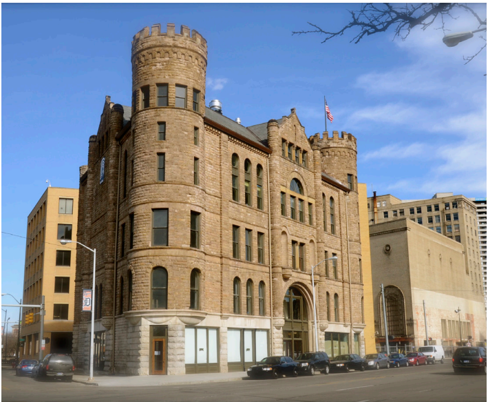
Grand Army of the Republic Building
