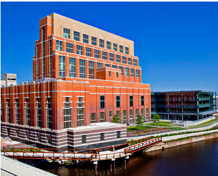
Ottawa Street Power Station, Lansing, MI
