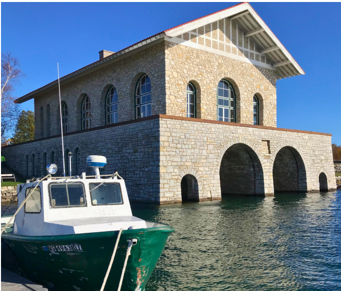
Rock Island Historic Boathouse Restoration
