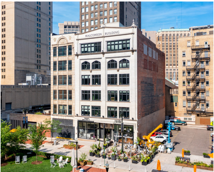
Malcomson Building, Detroit, MI
