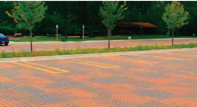
Permeable pavement parking lot infiltrates rainwater where it falls.
